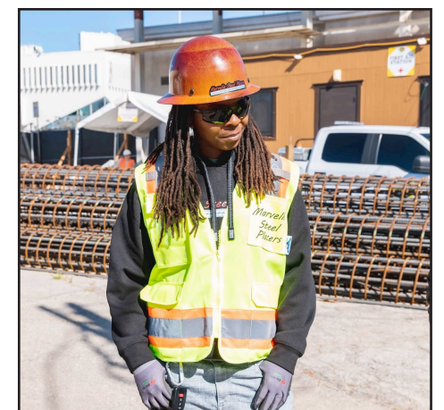
Pruitt oversees the unloading of rebar at the future site of Destination Crenshaw’s anchor attraction, Sankofa Park.
